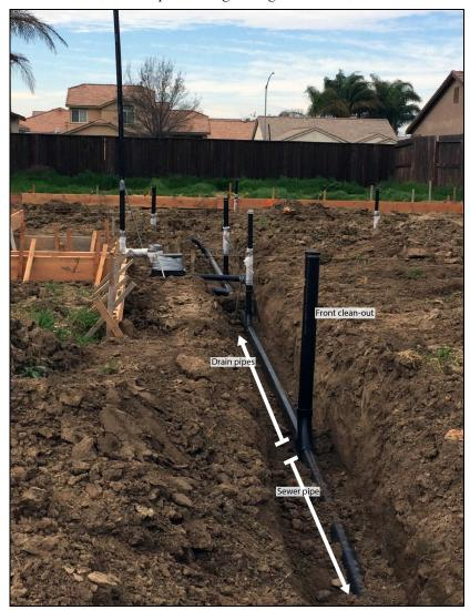
IDENTIFYING DRAIN PIPES FROM SEWER PIPI
