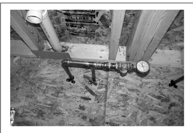
Testing with air is not permitted on plastic piping systems because of the hazards of a sudden release of energy, which could cause a separated piece of piping or a fitting to become a projectile causing serious injury.
